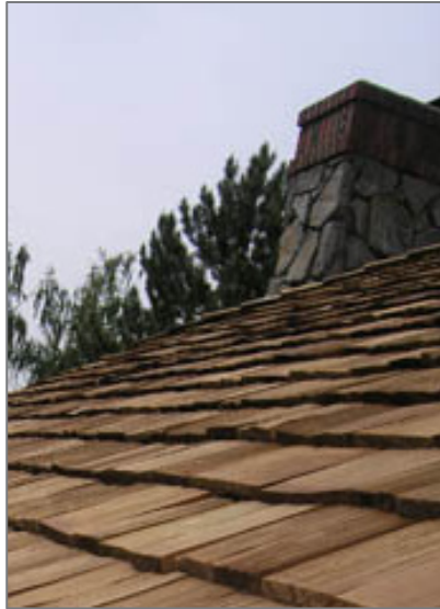
Wood shingle roof Courtesy of Gutter Glove
