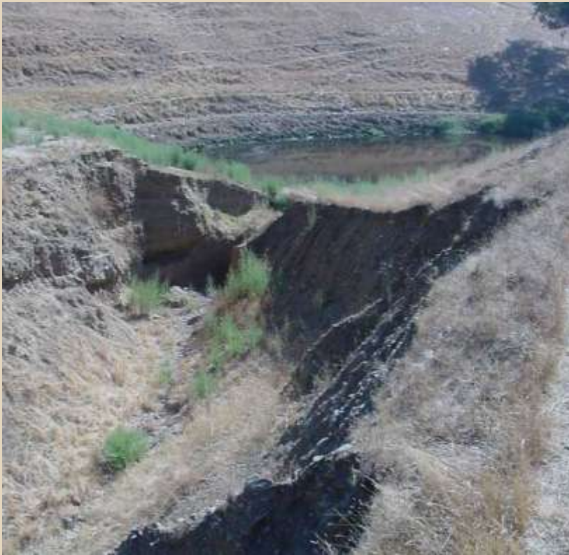
Spillway Erosion
