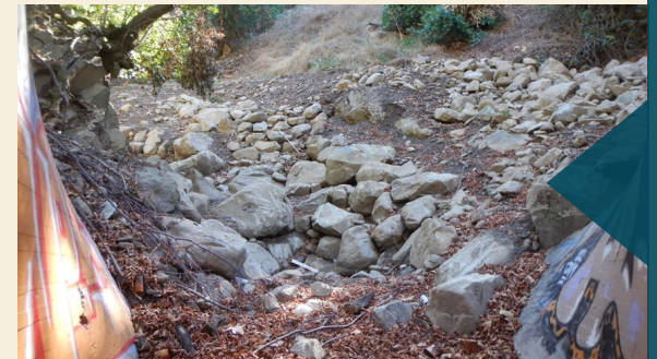
The boulder jam was removed and the channel regraded into a step-pool morphology
