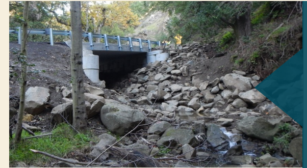
The bridge replacement and regraded channel with step pools improve passage conditions
