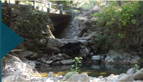
The slope of the culvert combined with the perched outlet was a significant barrier to fish passage
