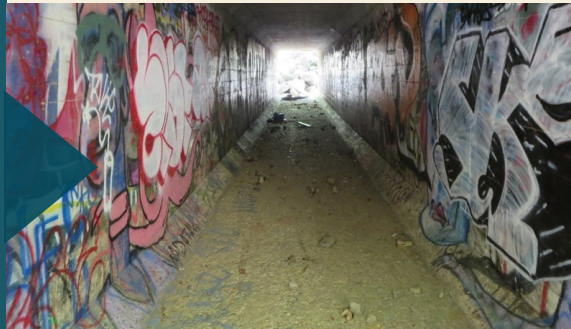
The old culvert conditions produced insufficient water depths and high water velocities limiting fish passage
