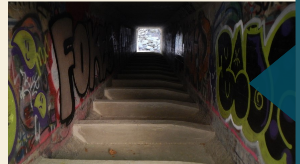
Baffles were added to retrofit the culvert to increase water depth and decrease water velocities within the culvert
