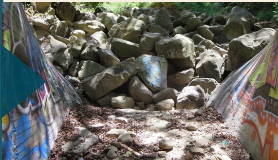
The boulder jam at the inlet of the culvert served as a full passage barrier within the stream
