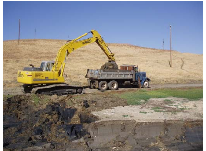
Livestock pond being desilted to improve habitat for California Red-legged Frog.
