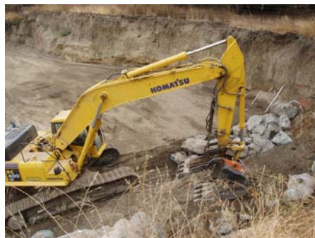
Left: Rock barb construction at the Arroyo de la Laguna Right: Western pond turtle, a California species of concern, found during construction at the Arroyo de la Laguna.
