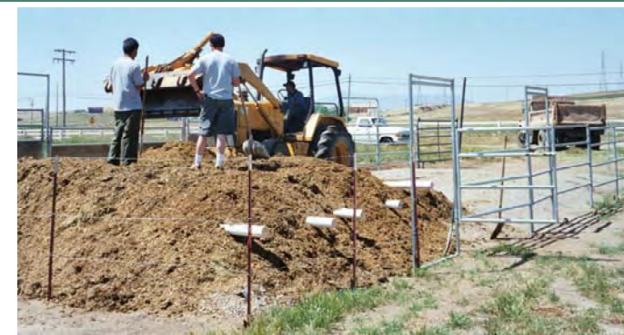
Above: Composting is done on a pad comprised of an impervious geofabric liner sandwiched between two 6 inch layers of crushed rock that has been compacted by a roller. This prevents drainage from the pile from leaching into the soil below the pad. Below: Manure is loaded on top of perforated PVC pipes which allows air to circulate through the pile. This is a cost efficient method for aerating the manure because the pile does not need to be turned. The pile is covered by a breathable tarp when needed to enhance composting and to shed excess moisture.
