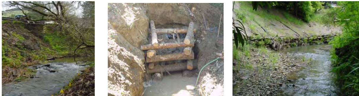
Left: This site suffered from severe erosion. Invasive weeds like cape ivy and periwinkle crowded out local native species. Center: The log crib structure consisted of non-native eucalyptus trees which had been removed from the site. Right: Once the structures were in place, soil was added on top and covered with coir fabric and a native grass seed mix. Native shrubs and trees will develop extensive root systems that will keep the soil in place once the structures decompose after 20-30 years.
