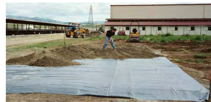
Above: Composting is done on a pad comprised of an impervious geofabric liner sandwiched between two 6 inch layers of crushed rock that has been compacted by a roller. This prevents drainage from the pile from leaching into the soil below the pad. Below: Manure is loaded on top of perforated PVC pipes which allows air to circulate through the pile. This is a cost efficient method for aerating the manure because the pile does not need to be turned. The pile is covered by a breathable tarp when needed to enhance composting and to shed excess moisture.
