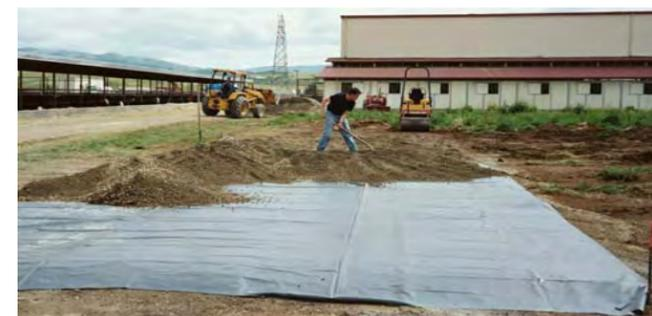
**Above:** Composting is done on a pad comprised of an impervious geofabric liner sandwiched between two 6 inch layers of crushed rock that has been compacted by a roller. This prevents drainage from the pile from leaching into the soil below the pad.
