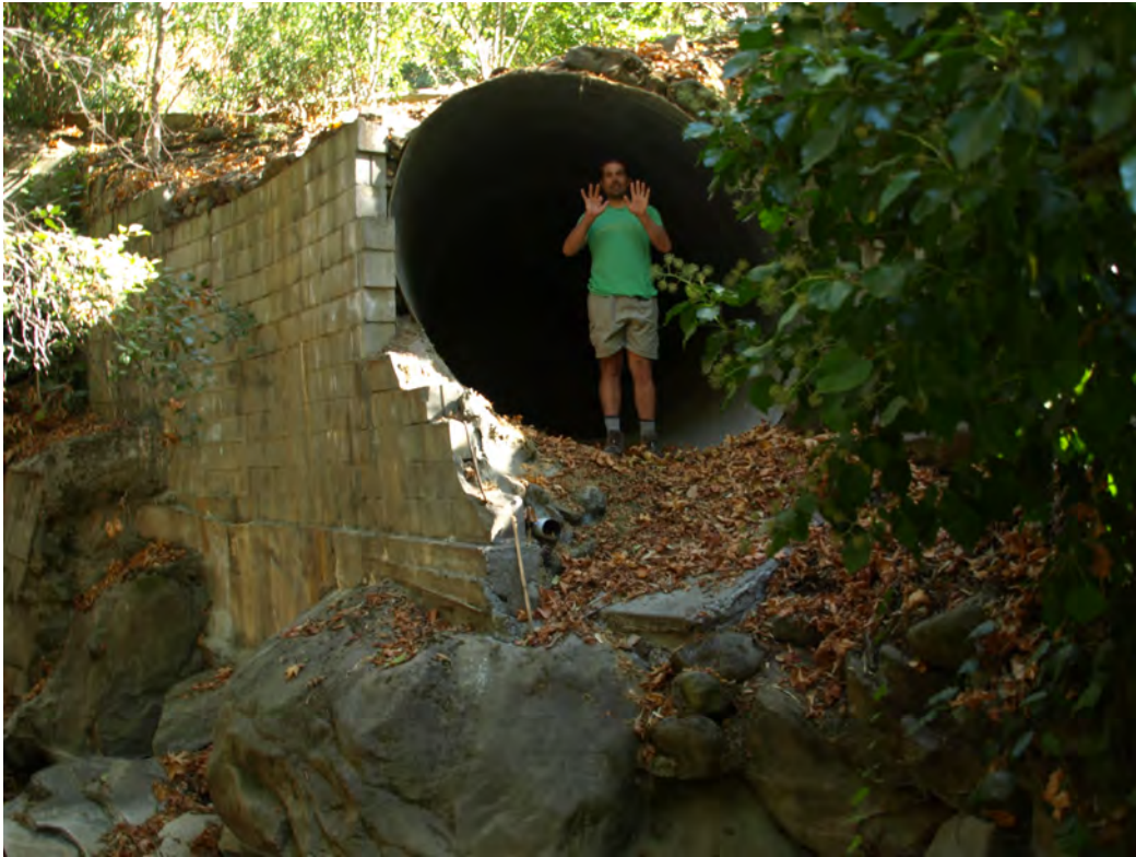
Photo 3. Culvert at Palomares Road MM 9.15
