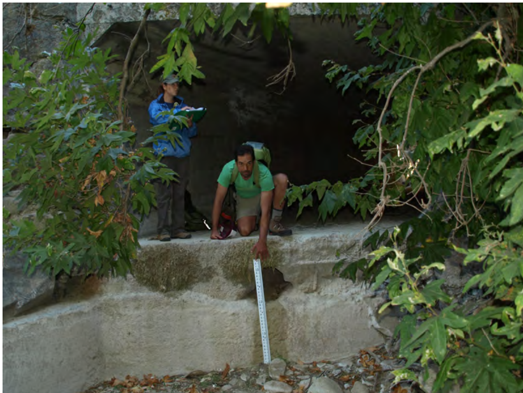
Photo 4. Stonybrook Creek culvert at Niles Canyon Road facing upstream.
