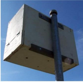
*Mounting by welding piece of angle iron*
