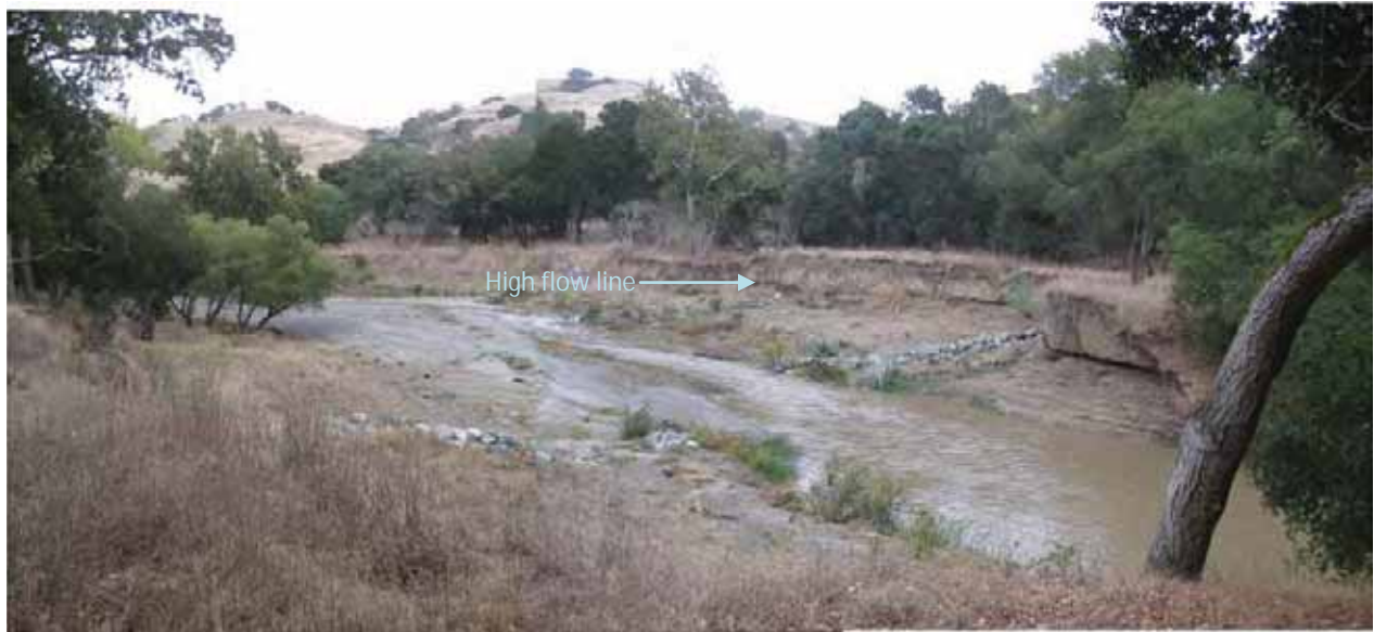
October 2009: Site After 10-13-2009 Storm Event (provisionally 6,600 cfs, later lowered)
