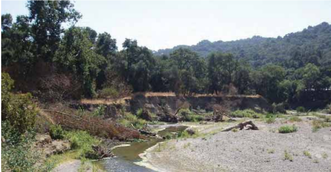
August 2006 Photo Monitoring Point 3
