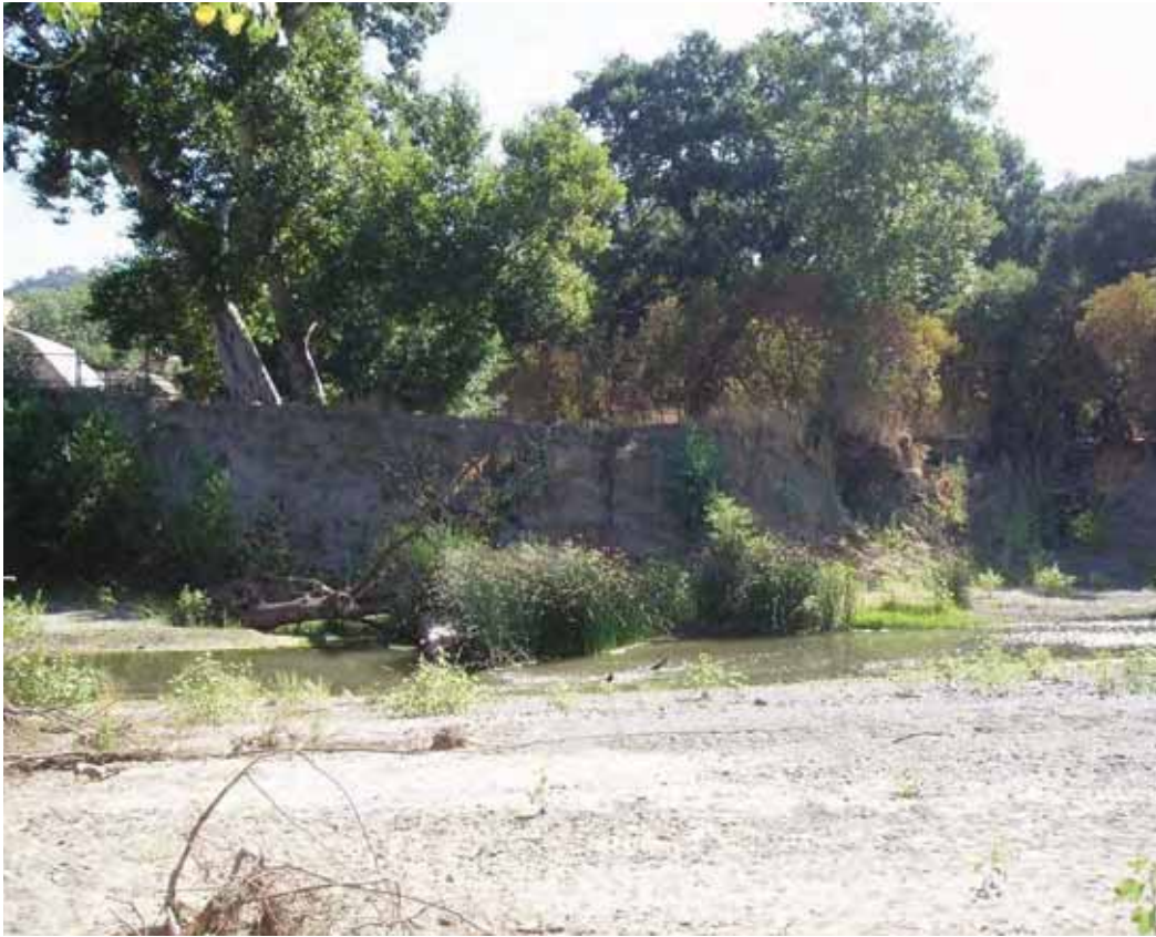
August 2006 Photo Monitoring Point 2
