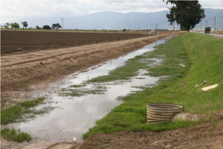
Figure 8. Shallow retention basins can infiltrate run-off from agricultural fields before it flows offsite
