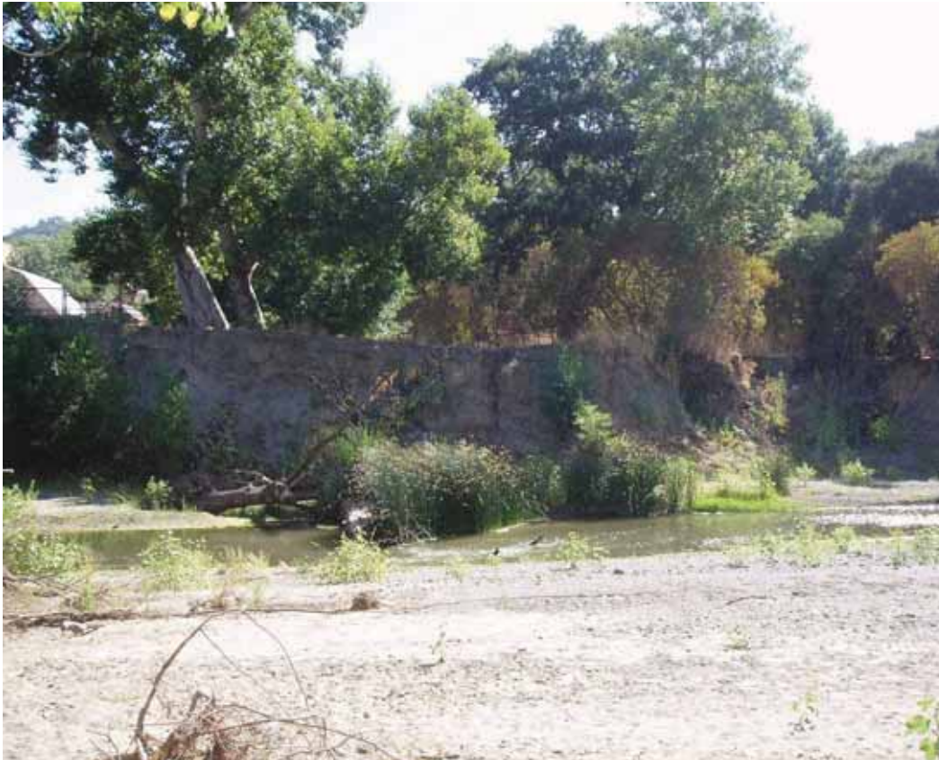
August 2006 Photo Monitoring Point 2
