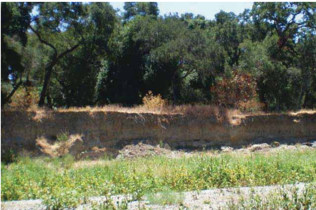
August 2008 Photo Monitoring Point 7
