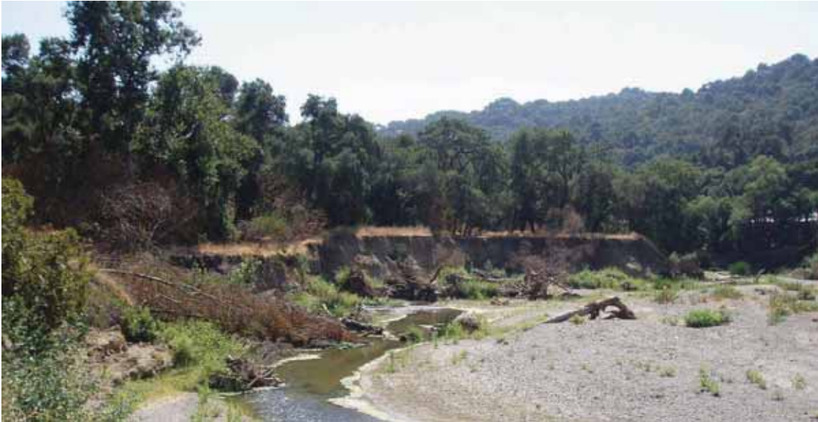
August 2006 Photo Monitoring Point 3
